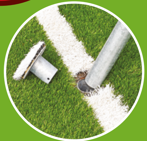
The sockets are hidden under caps
